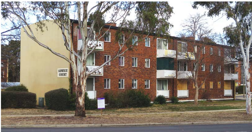
One of the blocks of the Stuart Flats (top) and Gowrie Court (bottom). Both complexes, built in 1959, are scheduled for demolition.
