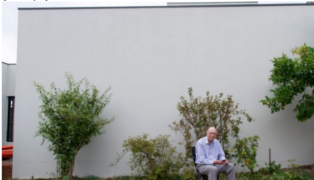
The 4.3 m high wall on the southern boundary of 16 Landsborough Street. It has severely restricted solar access to the neighbour's house (Image courtesy Fairfax Media).
