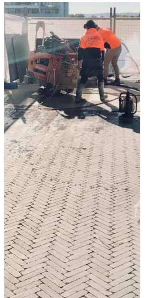
Dockside laneway during rain with water pooling in the paving recess/ Workmen repairing the part of the slab beyond the paving which is the most affected
